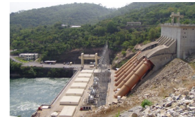
NODE A – GENERATOR (G1)
